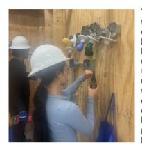
This week, students were introduced to a hands-on project involving four different lights powered by multiple light switches. The students learned how to properly connect the wires, using hot, ground, and neutral wires, to configure different light switch units. Towards the end of the week, the students got to experience using different power tools to cut and bend conduit. On Friday, they began the book portion of Lift Training and practiced on the scissor and boom lifts.
