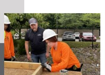
Youth creating forms, cutting wood and leveling the materials with a laser level and surveying equipment to prep for next week where they will be pouring multiple cement squares and learning how to use a skid steer.
